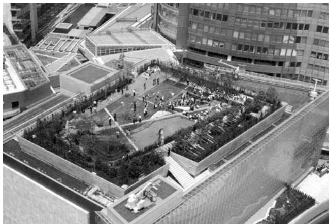
Figure C.30 A 'sky garden' at Roppongi Hills, Tokyo. (Source: Mori Building Co., Ltd.)
